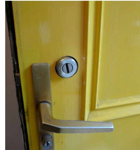
Outside View Front Door with new Mottura Key plus Key
